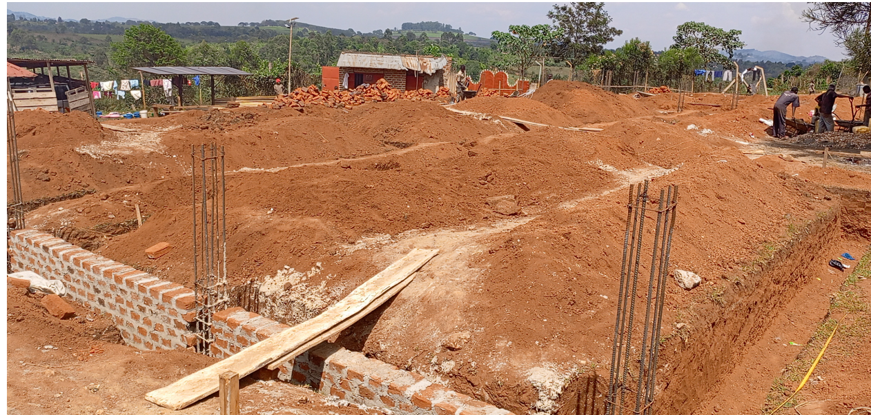
Dormitory under construction
